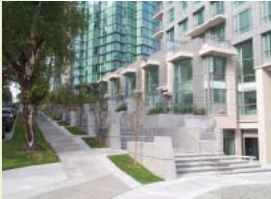
“Classico” rowhouses and public realm treatment enhance pedestrian scale on Jervis Street
