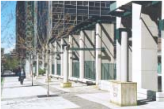
Colonnade frames the green court of “Venus” development on West Georgia Street
