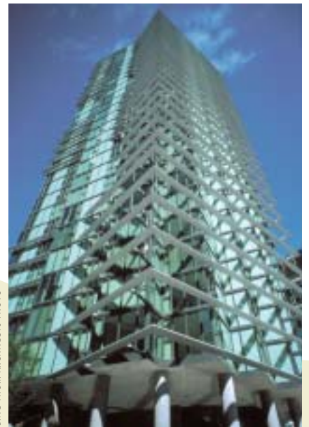
The 'brise-soleil' treatment of "The Pointe" tower references the West Georgia Street grid
