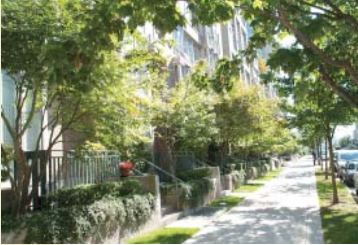
Marinaside Crescent, lined with townhouses and now maturing landscape, has achieved intended domesticity
