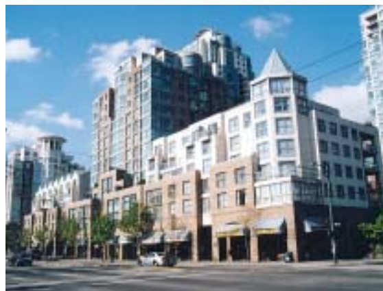
Streetwall massing on Main Street incorporating groundfloor retail with market and non-market housing above
