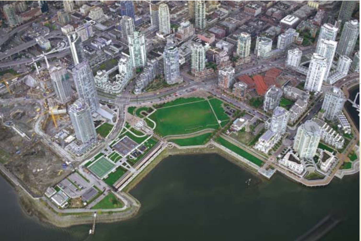
Beach Neighbourhood (left) under construction and Roundhouse Neighbourhood (right) frame David Lam Park (2003)
